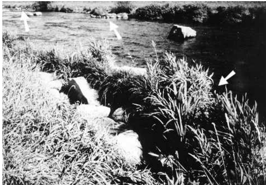
Figure 22. Photo of coir geotextile roll and rocks with wetland plants serving as a deflection system and providing aquatic habitat on a German stream. Note that two can be seen on the opposite bank also. (Photo courtesy of Bestmann Ingenieurbiologie, Wedel, Germany)
