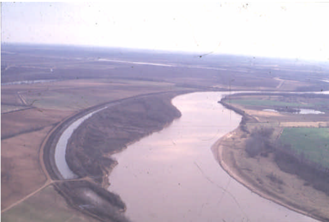
Figure 7.2 Aerial View of Trenchfill Revetment With Foreshore Material Still in Place
