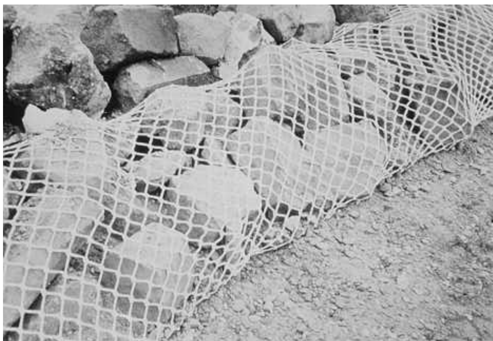
Figure 11. Rock roll used as toe protection on a bioengineering project, Rhine River, Germany, in the city of Dusseldorf.
