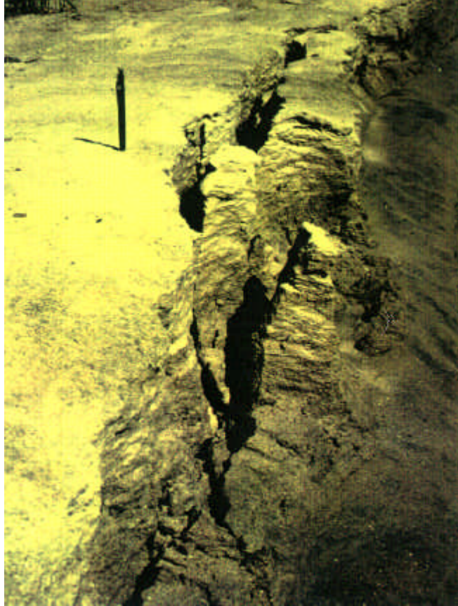
Figure 2.26 Soil Fall
