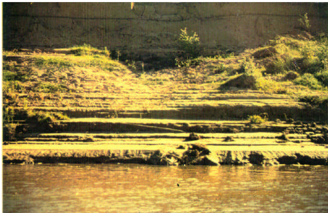
Figure 2.24 Erosion Generated by Wind Waves
