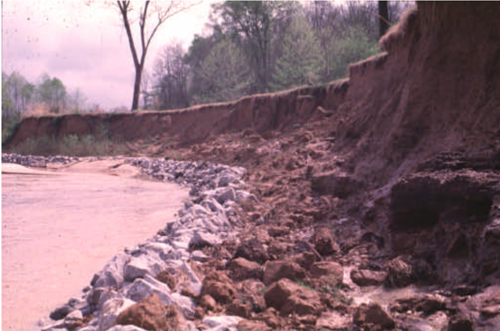
(a) One Ton Per Foot Immediately After Construction
