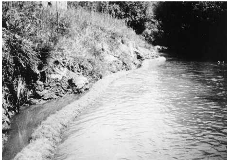
Figure 24a. Coir geotextile roll being installed along a streambank in Germany.
