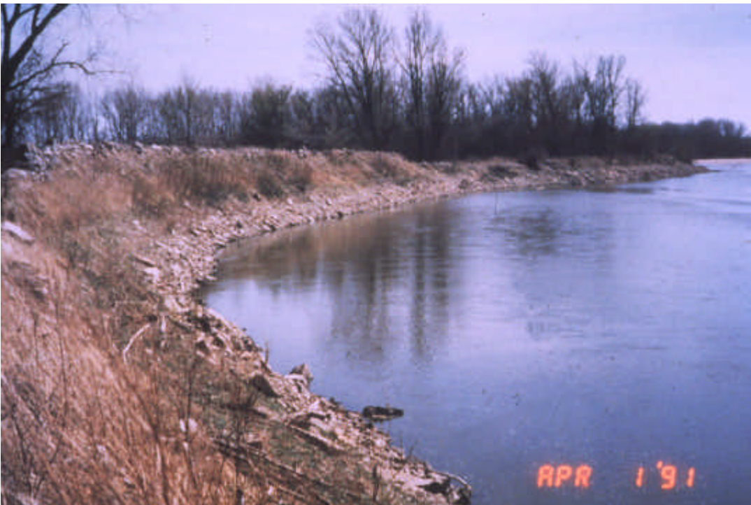
Figure 7.6 Launched Windrow Rock
