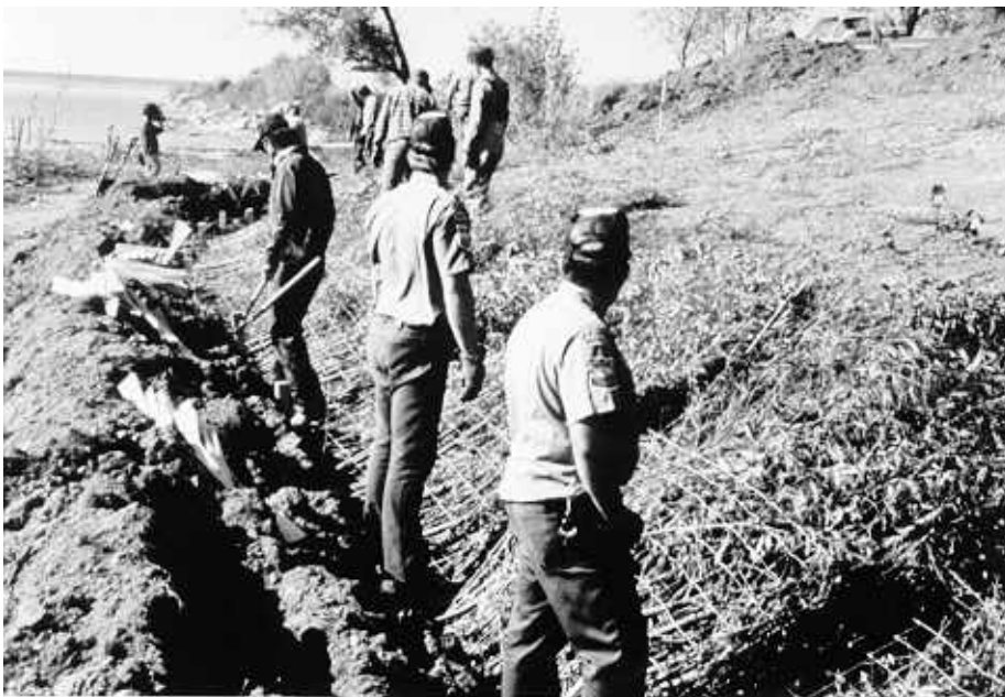
Figure 27b. Placing woven wire over the willow brush.
