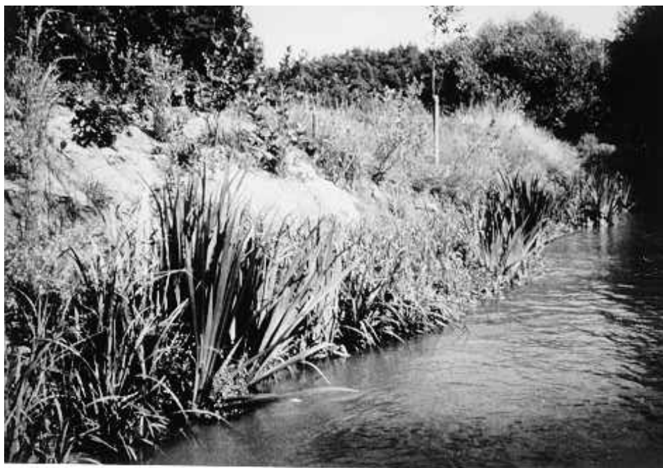
Figure 24b. Coir roll a month or so after planting.
