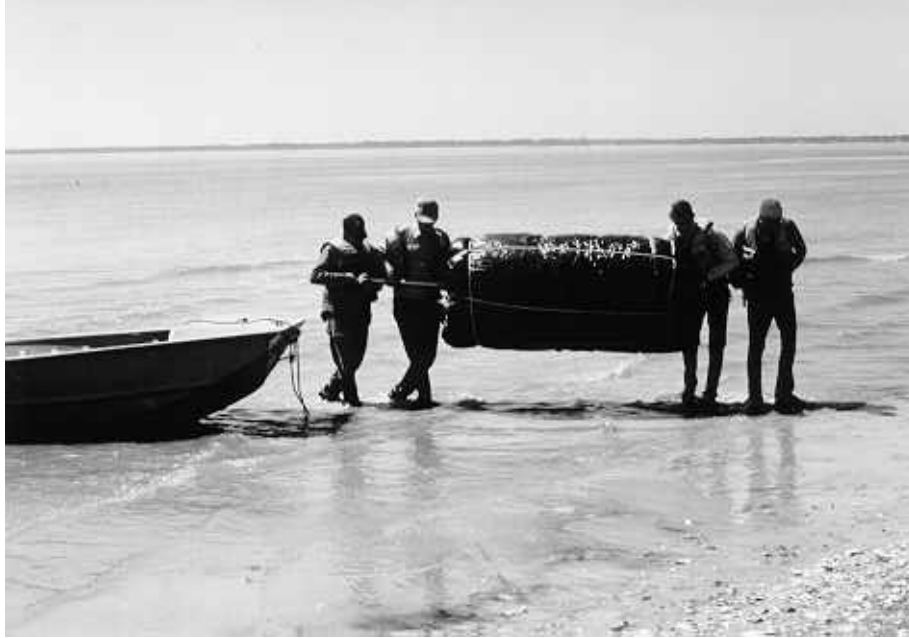
Figure 25c. Coir geotextile mat in a roll planted with emergent aquatic plants being carried to the planting site.
