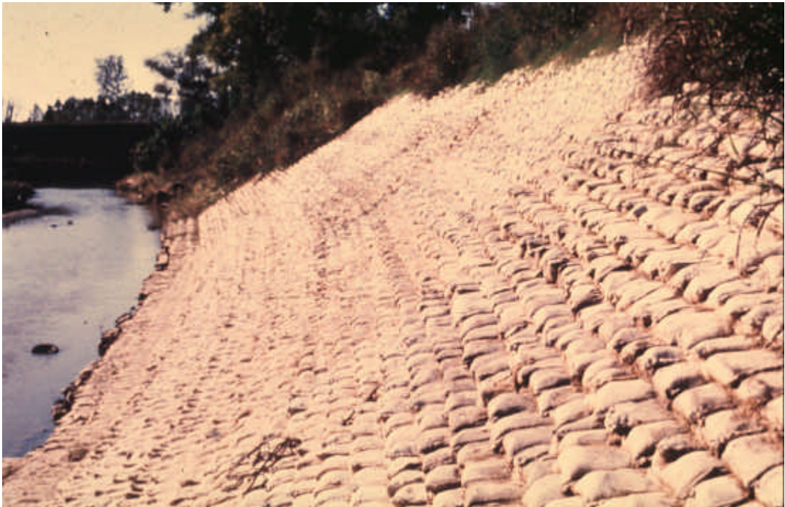
Figure 7.12 Typical Sack Revetment
