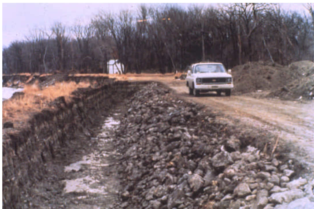
Figure 7.5 Placement of Windrow Rock in Excavated Trench on Top Bank
