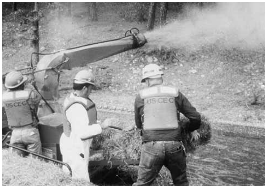
Figure 42. Hydroseeding and mulching operation from a barge.
