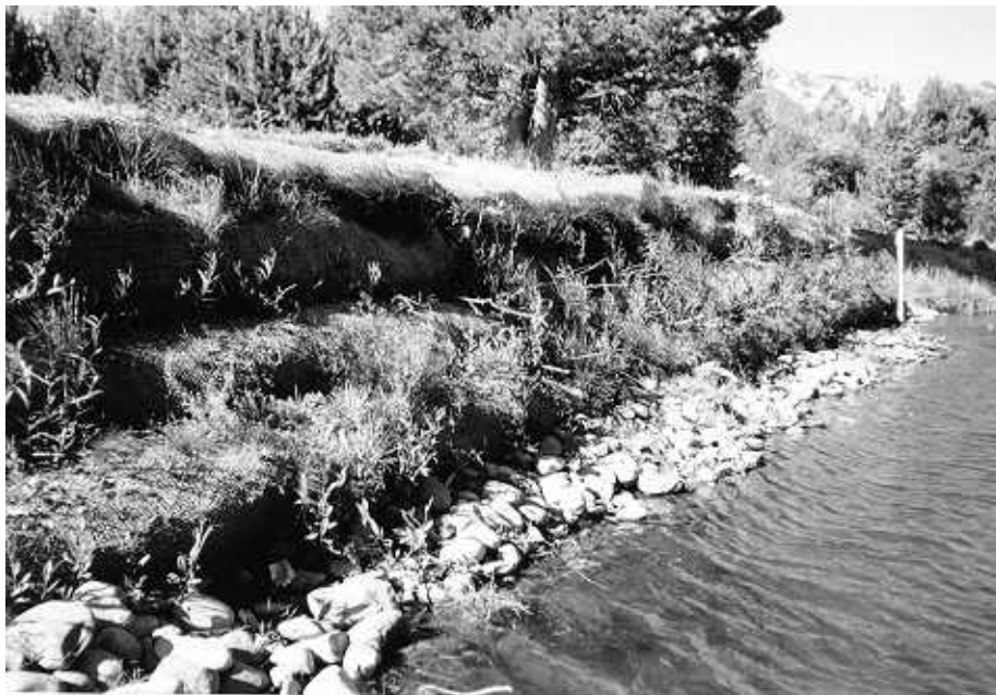
Figure 33. Vegetative geogrid in July 1995, after two growing seasons and an estimated 5-yr flood during the spring of 1995. Note that live willow whips which were placed between the layers of COIR fabric are sprouting and spreading. (Photo courtesy of Ms. Catherine McDonald, Calif. State Parks)
