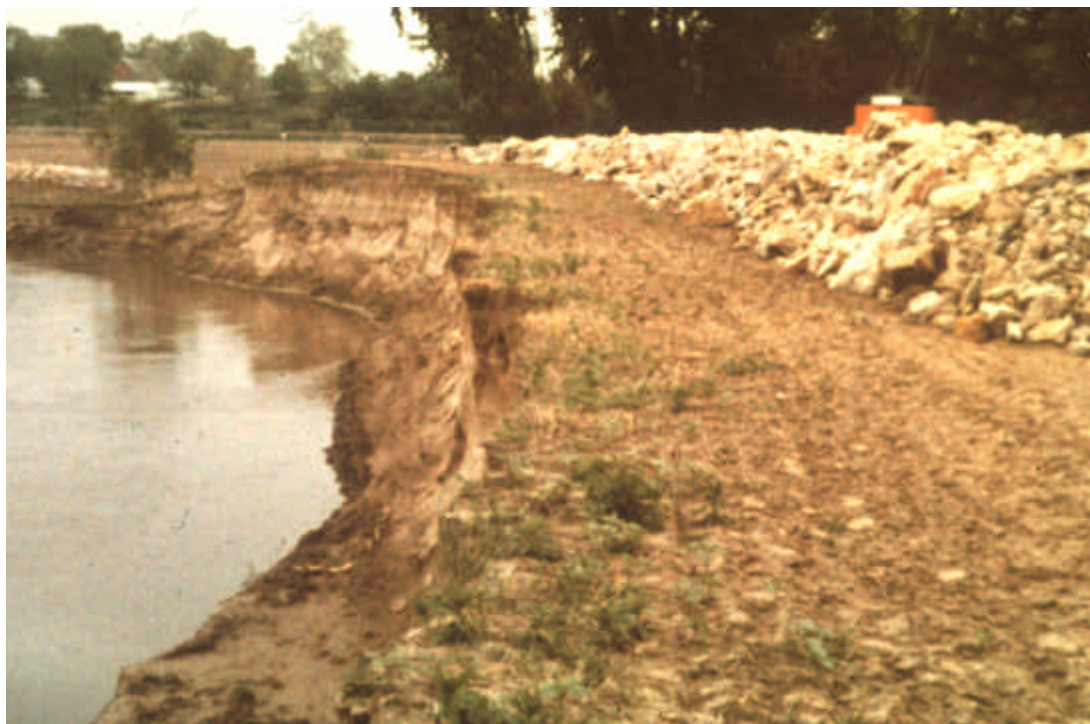
Figure 7.4 Conventional Windrow Placed on Top Bank
