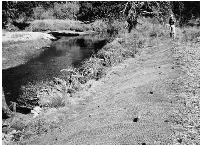
Figure 20. Root wads soon after installation on the Upper Truckee River, California, near South Lake Tahoe. The voids within and between the root wads are filled with a soil mix and planted with live, vegetative clumps or root pads, such as willow.
