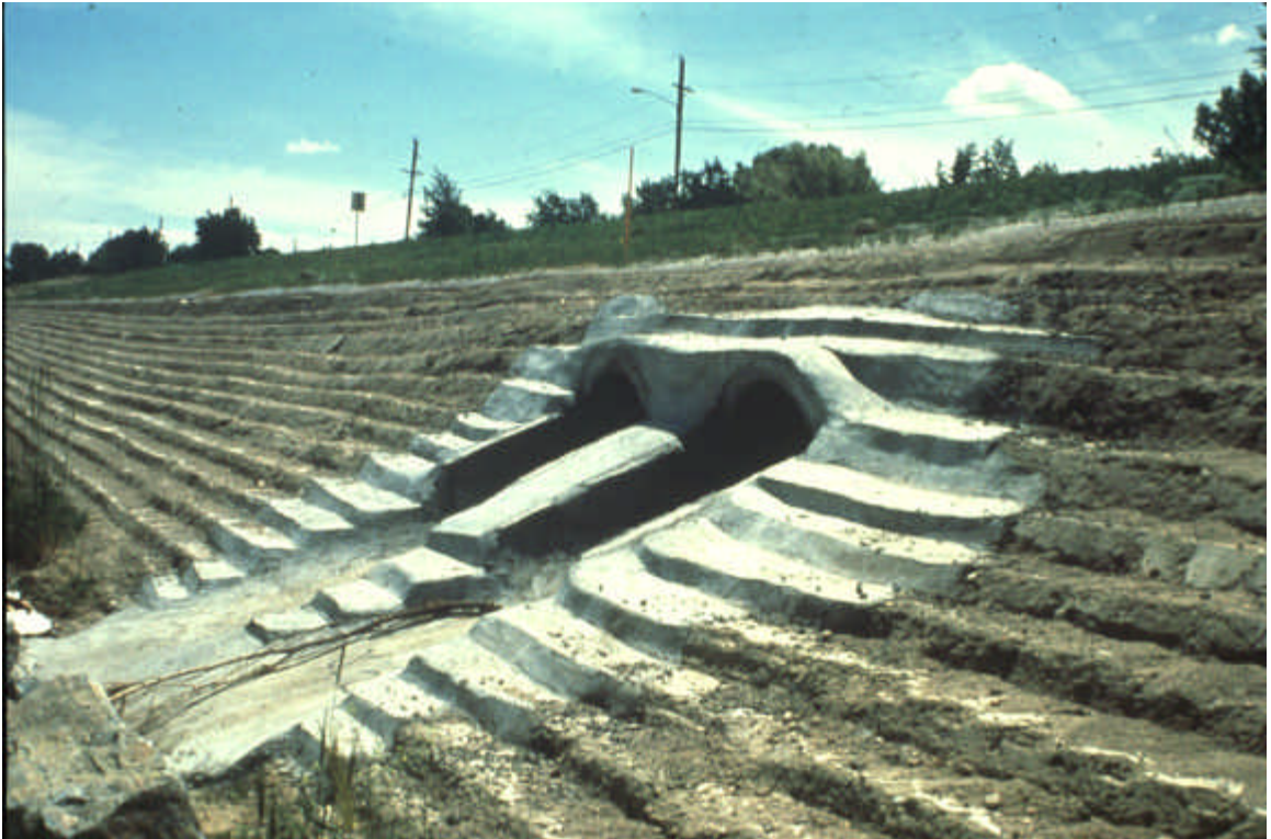
Figure 7.13 Typical Soil Cement Application
