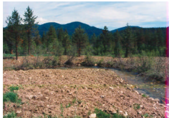
Figure 1. Rootwad composites after installation along a Montana stream
