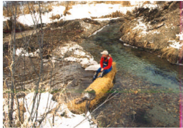
Figure 10. Temporary water diversion through point bar
