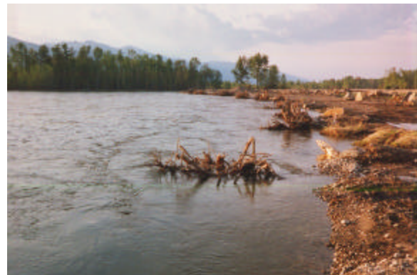
Figure 2. Project is not complete, but illustrates displacement of the current line away from the streambank (courtesy of Water Consulting, Inc.)
