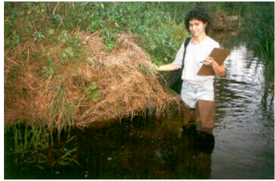
Figure 3. Rootwad composites can offer substantial habitat complexity. Prior to installation of rootwad composites, this streambank was raw and eroding
