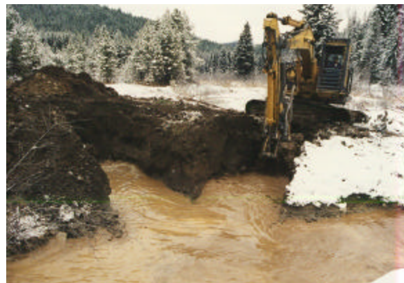
Figure 11. Trenches for rootwad bole and footer log
