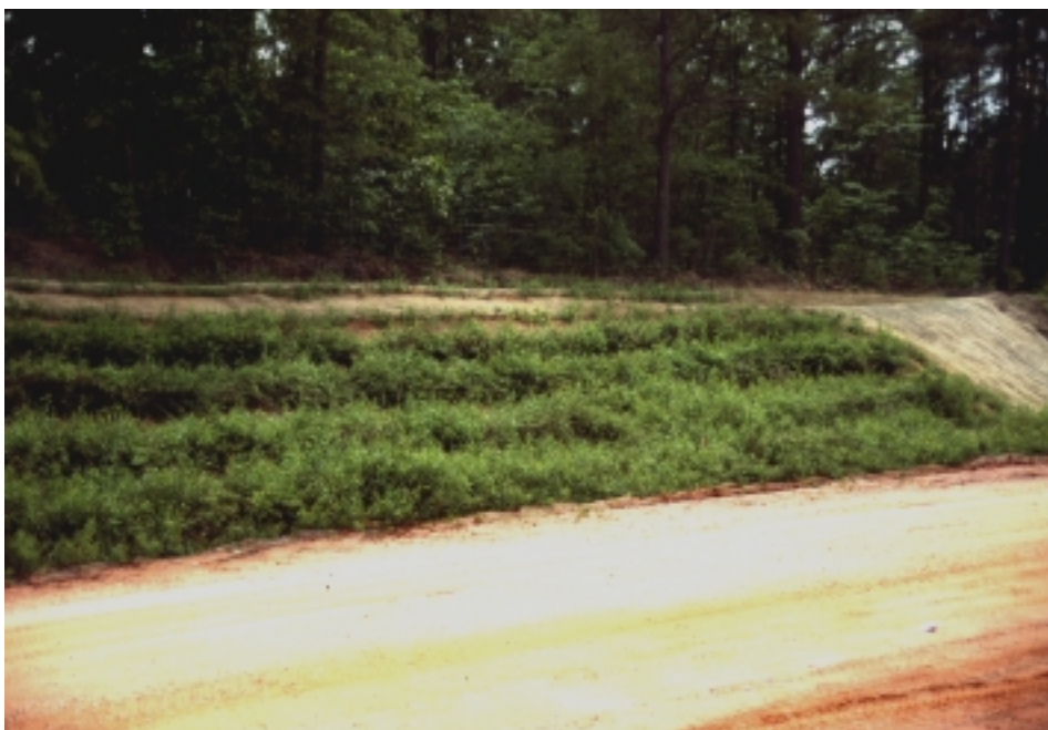
Figure 18-11b Two years after installation
