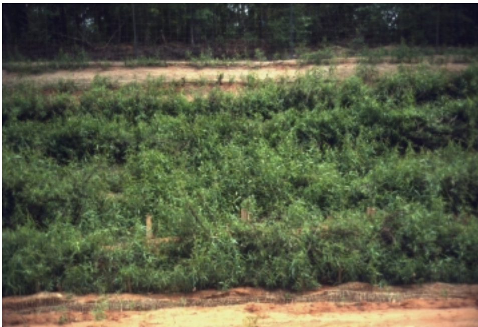
Figure 18-15b One year after installation
