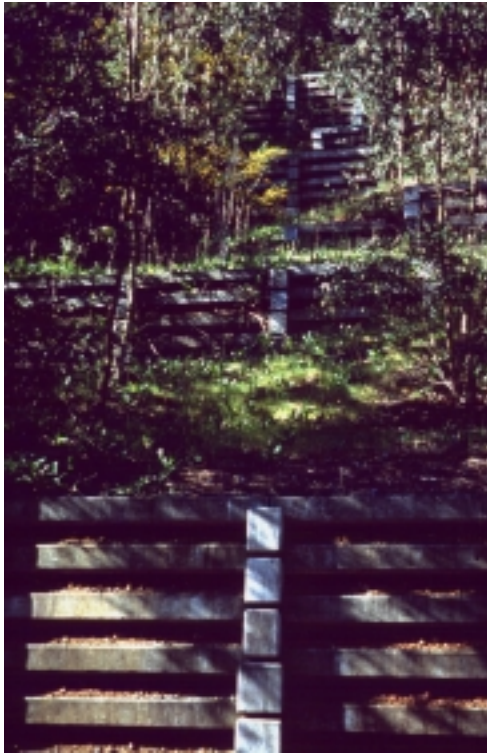
Figure 18-28b Open-front concrete cribwall with plantings in openings
