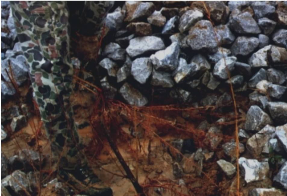
Figure 18-23a Root system 7 months after installation
