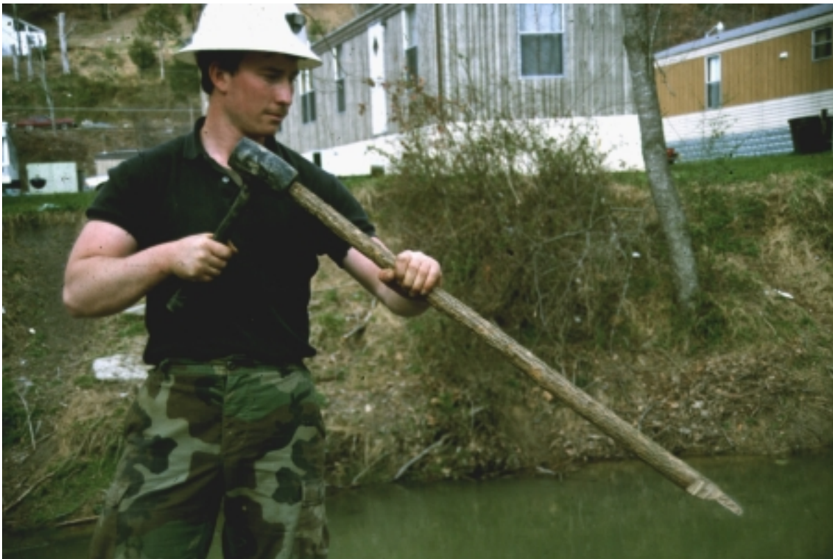
Figure 18-5 A prepared live stake (note angled basal end and flat top end) (Robbin B. Sotir & Associates photo)
