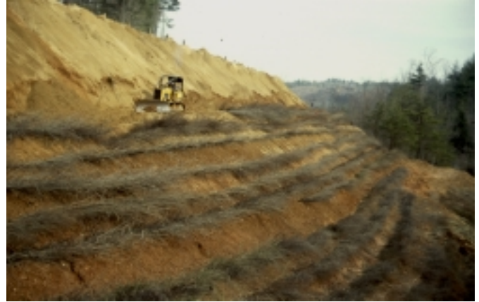
Figure 18-1b Measures being installed
