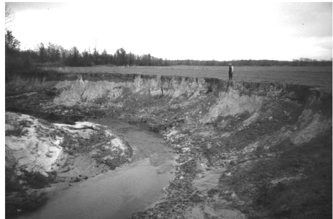
Figure 2. Bank erosion along study reach, 1999.
