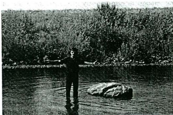
Figure 1. Invasion of Riprap Revetment by Pioneering Woody Species.
