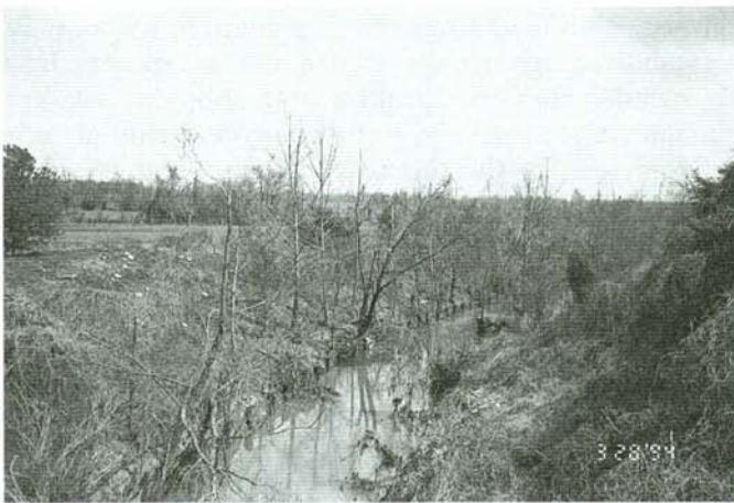
Figure 8. Site VTS2 13 Years After Construction. This photograph is taken from the same point as Figure 1. Schematic of design is shown in Figure 5.
