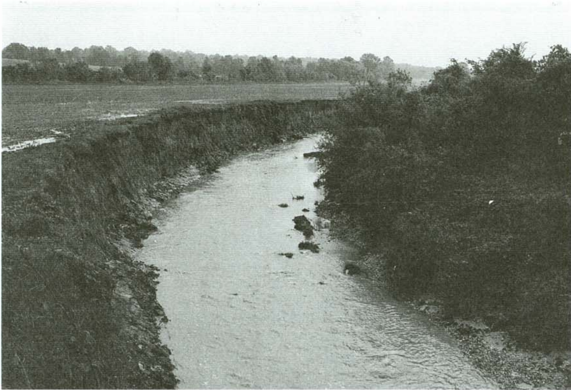
Figure 1. Erosion Triggered by Channel Erosion. Channel shown drains only 16 km 2 , but bank height is between 4 and 5 m. Photograph is looking upstream from downstream end of site VTS2.
