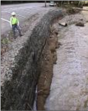
Photo 168. Receding storm runoff 1 Mar 2000 Looking downstream.
