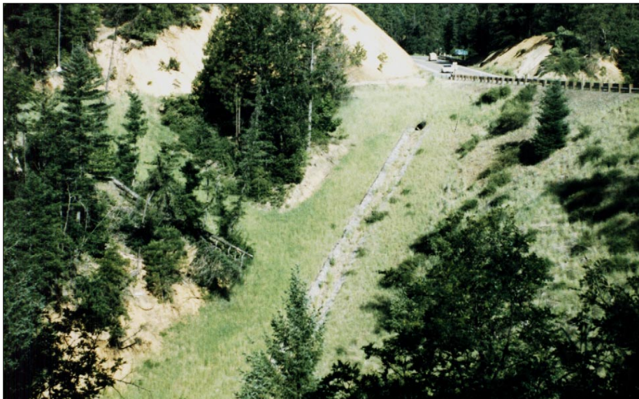
Photo 121. Same view as photos 119 and 120 after 6 wet seasons, 22 June 1993. Slopes OK.
