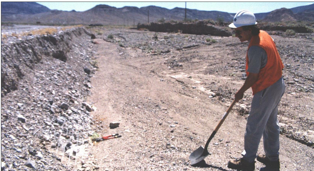
Photo 107. Collecting soil sample, looking upstream, easterly. Shovel at approximate edge of 3-foot by 3-foot counterfort (OK, buried). Flash flood impinged and combined with parallel flow, drainage paths visible from right to left and from left of center. Compare to photo 103.
