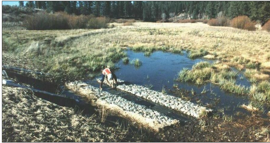
Photo 67. Author fastening test panels to gabion energy dissipater, 2 Nov 1989.
