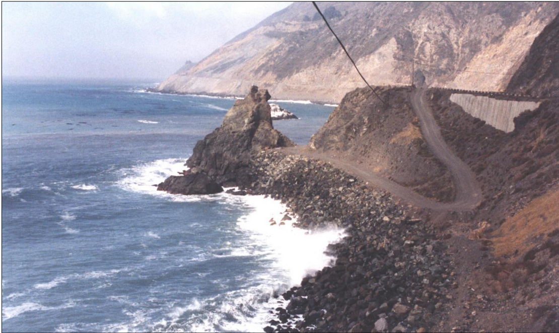
Photo 87. Normal high tide, waves break directly on south RSP, a deepwater revetment, looking northerly, mostly OK after 13 wet seasons, 4 Nov 1998. Nearly same cross-section as north RSP, except toe of PVC-coated gabion mattresses are at elevation 10 feet, 8-ton rock toe extends below mattresses. Duck Pond slide (Jan 1997) is bare land feature in far left background on point, more than 1 mile distant. Access to north RSP down steep grade from route 1, through rock cut, then to right.
