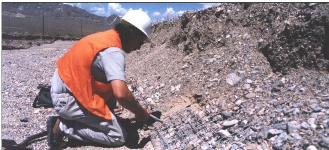
Photo 109. Repaired cut-out zone with interlocking fasteners and special long-handled pliers.
