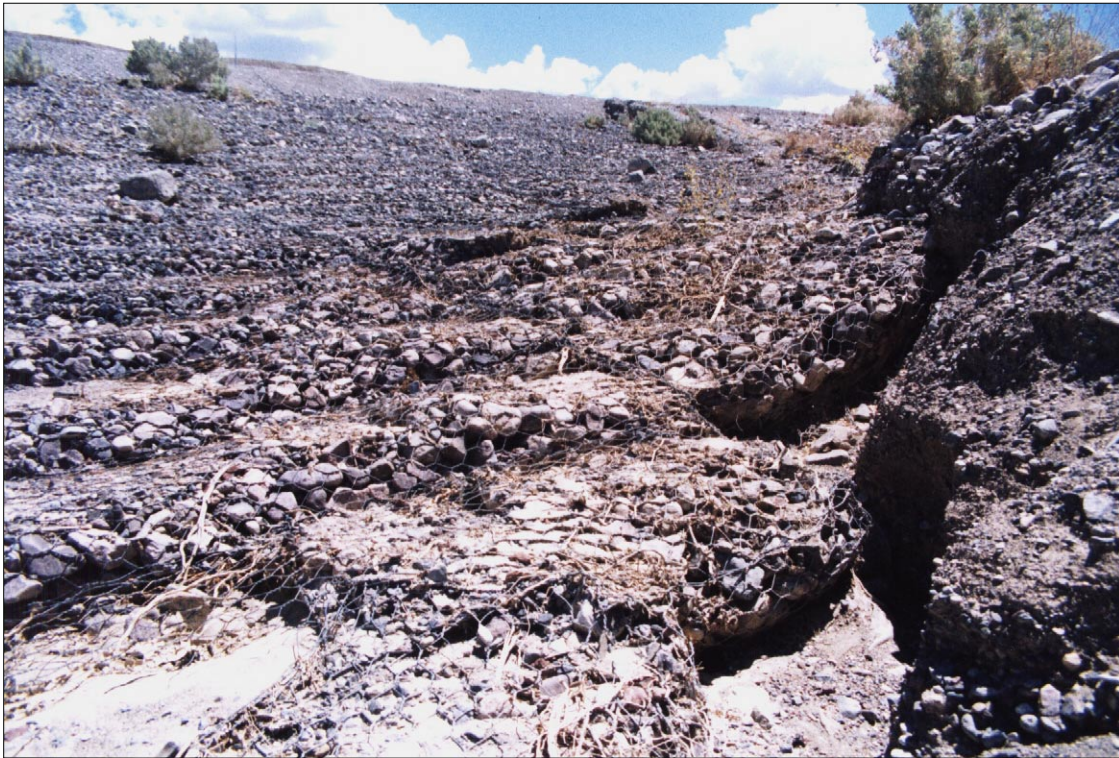
Photo 114. Gabion-protected slope is spillway-downdrain for flash floods, looking up-slope and upstream in Gower Wash (gully at right is seen on left in photo 112), 9 Jun 1998. Some lids failed due to abrasion by sand and gravel transported during floods. Brownish color is silt residue, and some rusted wires.
