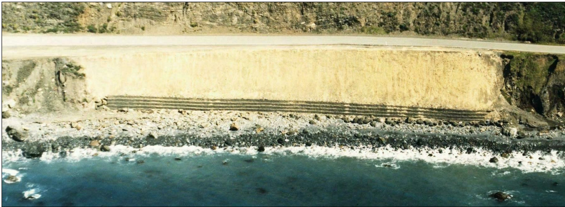
Photo 90. Oblique aerial view of south wall after about 1 wet season. 24 March 1986, looking easterly, post mile 7.7. Normal daily high tides reach about elevation 6 feet, rocky beach buffers wall from daily wave attack. During severe storms, waves reached top of wall, about elevation 25 feet, occasionally overtopping wall.
