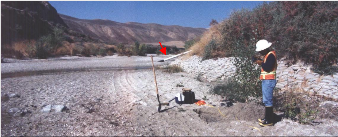
Photo 131. Found gabion check dam buried about 0.5 foot, looking upstream. Wire in very good condition after 2 wet seasons. Trickle flow meandered to opposite side of creek, soil was saturated. White-to-black natural gas pipe (arrow) exposed in degraded creek bed.
