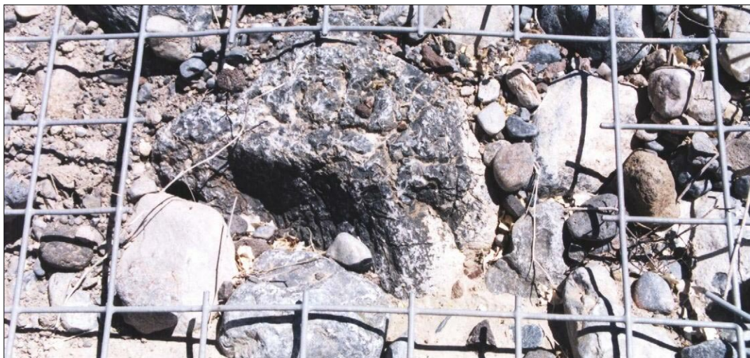
Photo 108. Removed sample from gabion mattress lid. Gray PVC-coated, 3" x 3" welded mesh.
