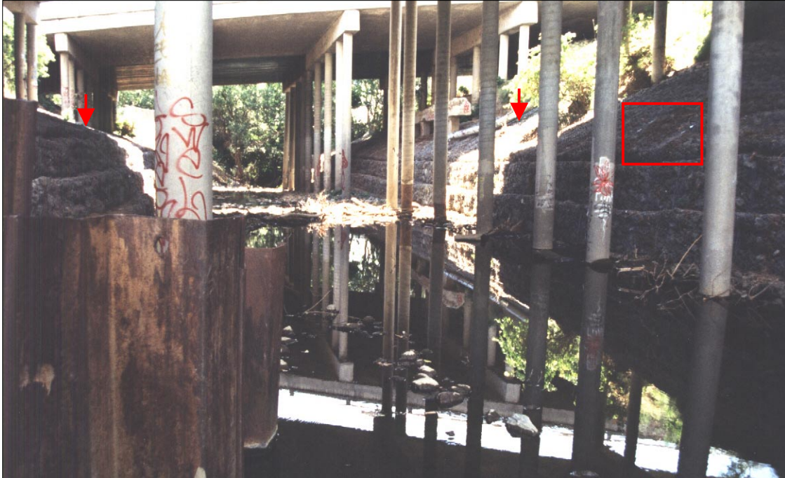
Photo 134. Looking downstream under bridges 23-0052 left and right, after one wet season.
