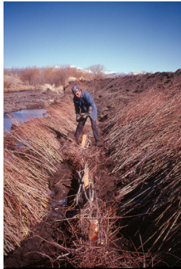
LLL-Reach A Project: During and After Construction of Live Siltation, Willow Wattle, and Brush Mattress
