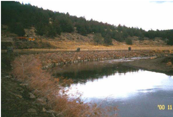
Bushey Project: Vegetated Riprap 1 month and 1.5 years after construction
