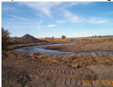
LLL-Reach B Project: Before, During and After Realignment and Installation of Brushlayering with Rock Toe
