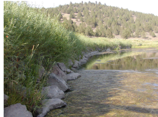
Bushey Project: Vegetated Riprap 1 month and 1.5 years after construction
