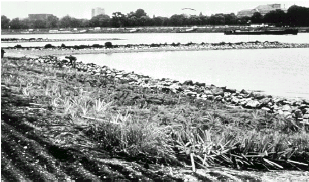
Figure 5.11. Large rock transverse dikes (photo courtesy of Bestmann GmbH, Wedel, Germany)
