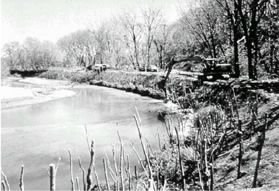
Figure 5.33. Work in progress
