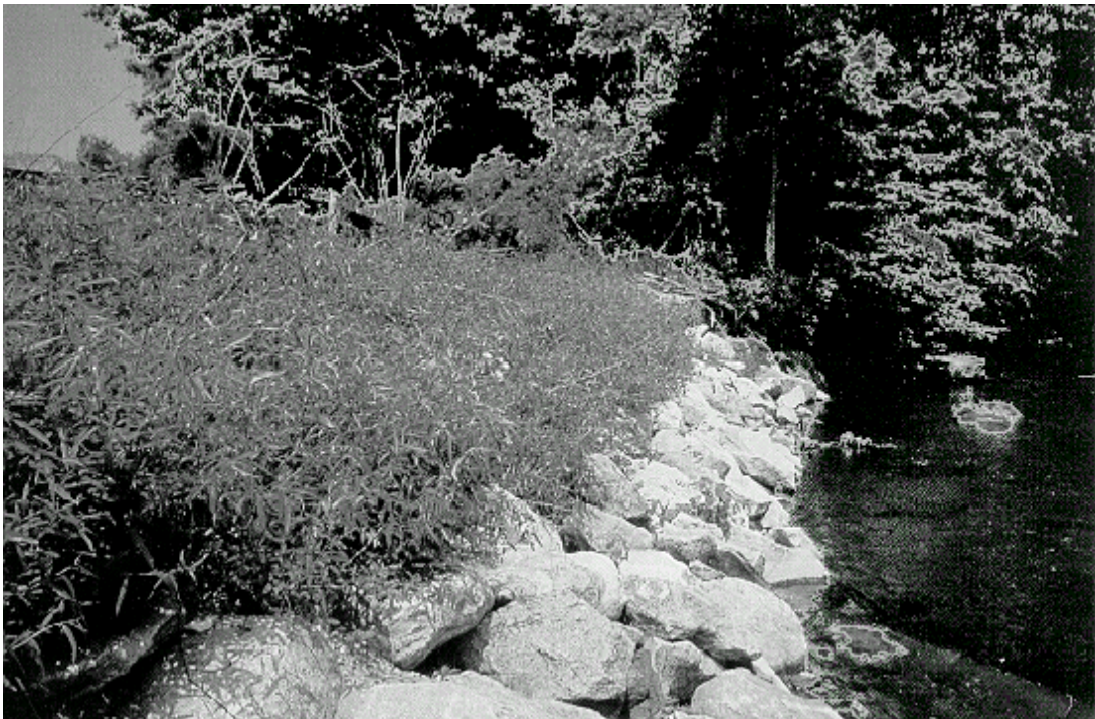
Figure 5.29. Brush layering or branch packing completed (Bowers 1992)
