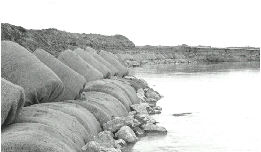
Figure 5.8. Rock toe with hay bale cylinders
