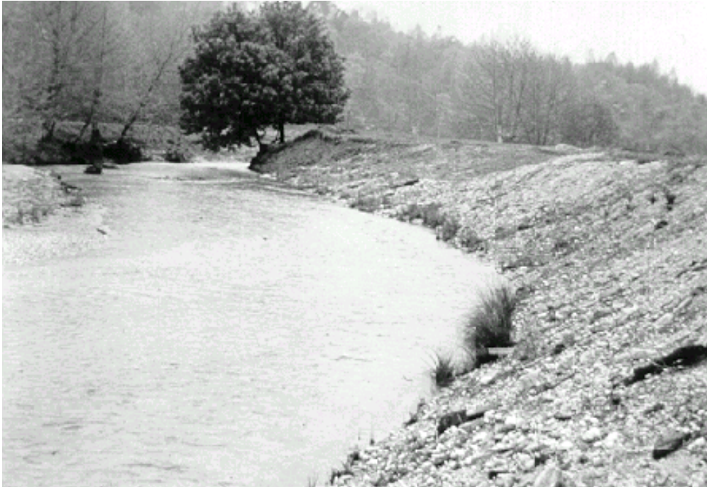
Figure 5.36b. Application of bankers and streamco willow cuttings, before
