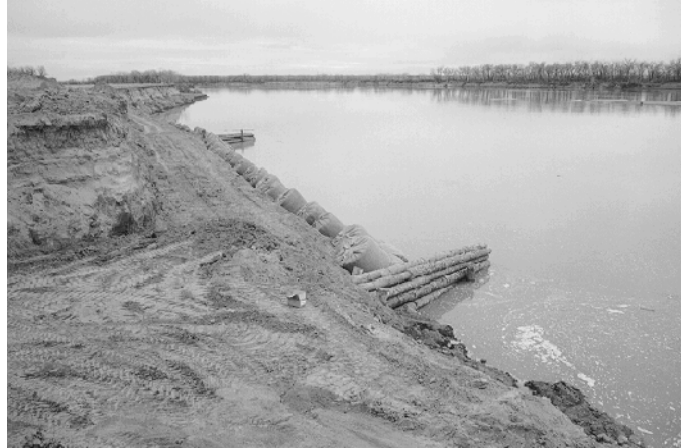
Figure 5.2. Cribbs serving as deflection structures
