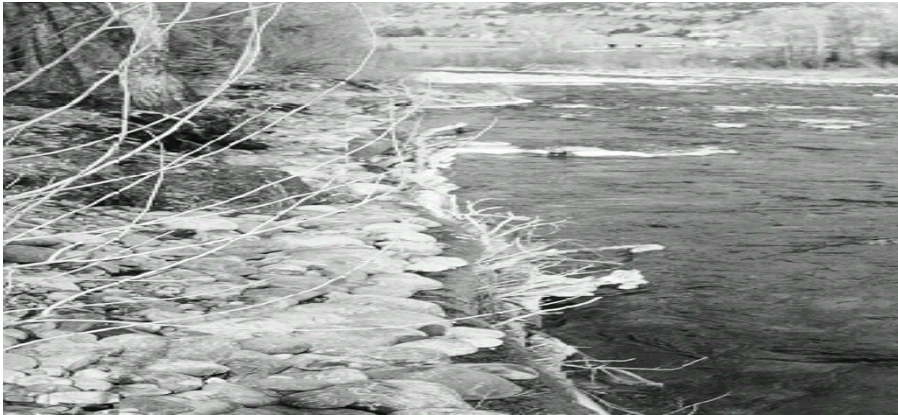
Figure 5.17. Installed log revetment
