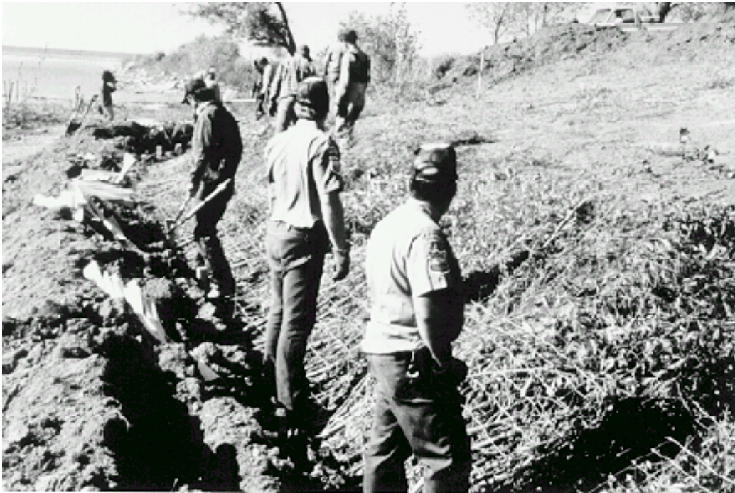
5.26b. Securing woven wire over a brushmattress
