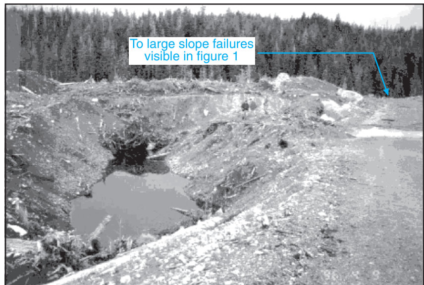
Figure 2. Flooded quarry above headwall of largest slide visible in figure 1. Immediately to the right of this photograph there was a second flooded quarry (see figure 1).
