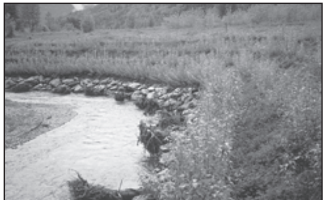
Figure 5. July 2000. Site B after two seasons' growth. Note elevated rootwads.
