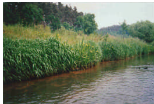
Figure 1. CGR after installation along a German stream (photo courtesy of Bestmann GmbH, Wedel, Germany)
