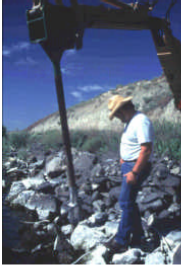
Figure 6. Stinger inserted into metal cap pushing willow post into rock (photo courtesy of Chris Hoag, NRCS)
