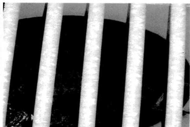
Riser chamber clear of sediment & trash
