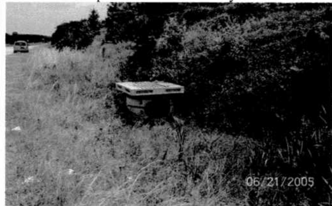
Clear & functional upper stage orifice
