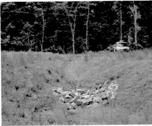
Stabilized conveyance channel into Basin
