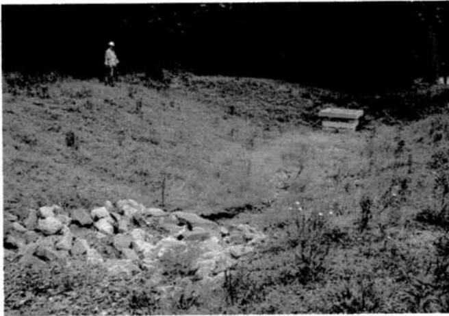
Well maintained and acceptable Basin embankment
