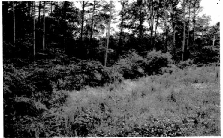
Basin embankment with woody vegetation of 0.5 to 2 inches
