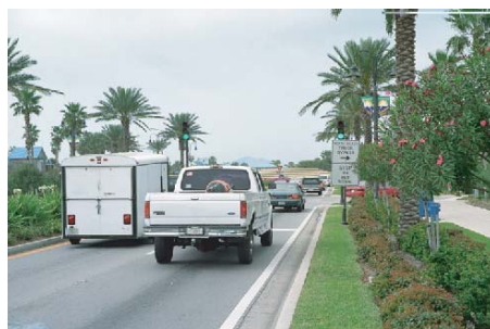
(a) Approach metering signal Clearwater, Florida
