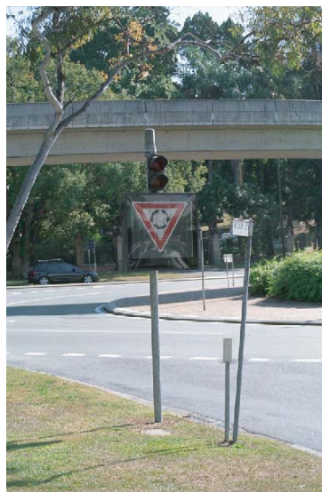
(c) Combination metering signal and changeable yield sign Brisbane, Queensland, Australia
