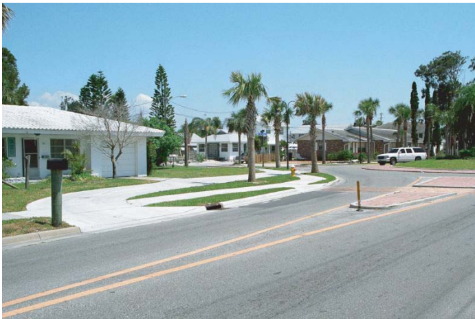
(c) Driveway reconfiguration (Clearwater, Florida)
