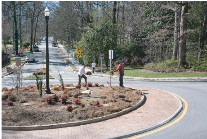
(a) Central island maintenance (Decatur, Georgia)
