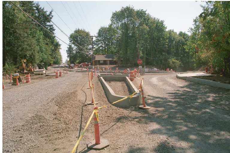
(a) Splitter island construction (Portland, Oregon)
