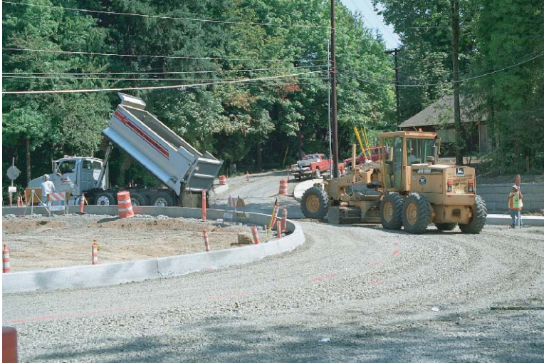
(b) Circulatory roadway sub-grade construction (Portland, Oregon)
