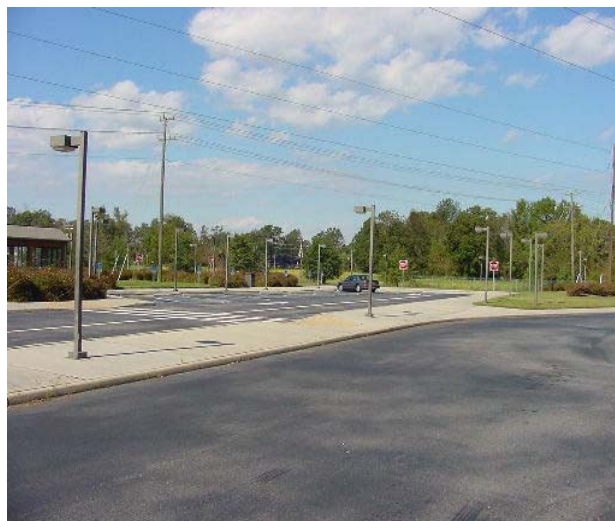
Figure 3-8: Lighting in the Kiss-N-Ride Area
