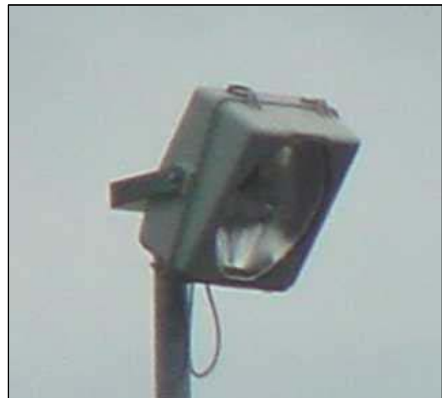
Figure 2-9: Offset Luminaire Note: VDOT lighting designs no longer use non-cutoff tilted luminaires.
