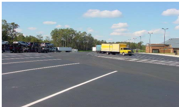
Figure 2-8: Truck and Camper Pavement Markings
