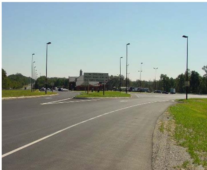
Figure 1-1: Rest Area TCD (Signing, Marking & Lighting)
