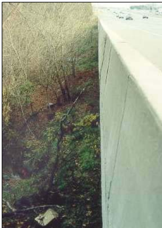
Figure 3-1: Difficult Terrain Features. 25-foot drop to ground level with steep grade.
