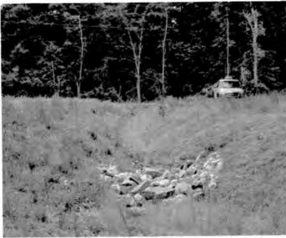
Stabilized conveyance channel into Basin
