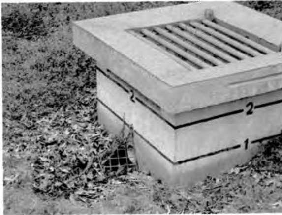
Clear low flow orifice w/ functional trashrack Low flow orifice blocked by trashrack
