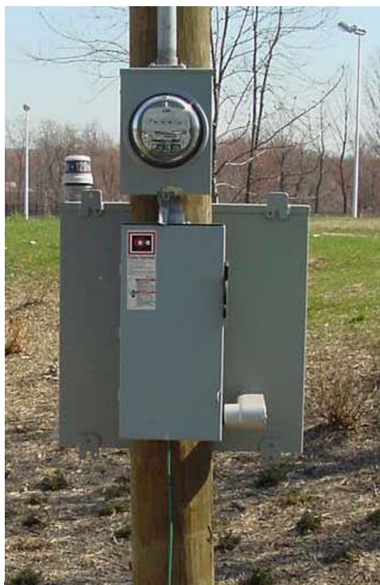
Figure 2-18: Standard VDOT SE-8 Type-A with CCW-C
