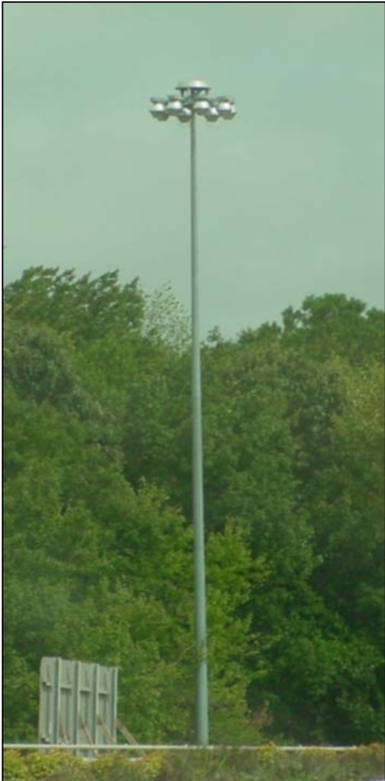
Figure 2-14: LP-3 High Mast Lighting Standard
