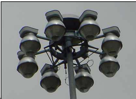
Figure 2-8: High Mast Luminaire Assembly
