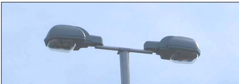
Figure 2-10: Dual Offset Luminaires
