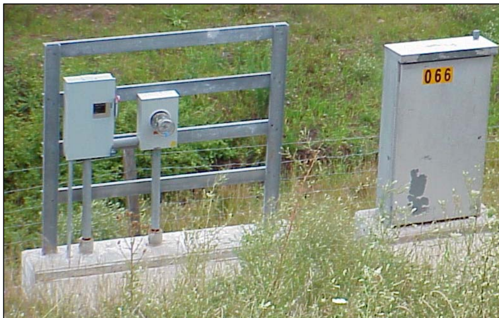
Figure 2-17: Standard VDOT SE-9 Type-A.
