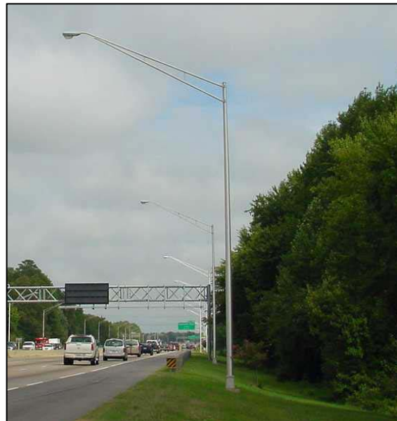
Figure 2-12: Conventional or Cobrahead Lighting Standard
