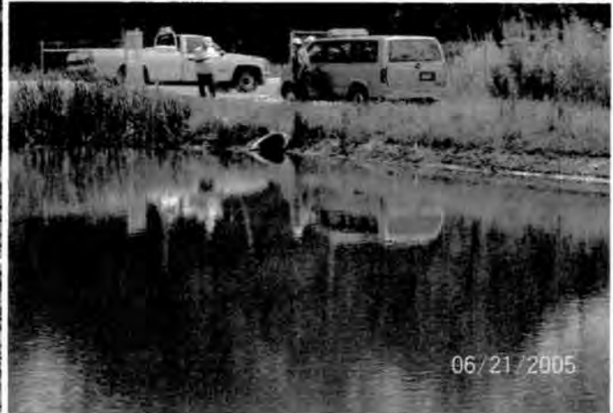
Principal spillway with pipe only, no structure
