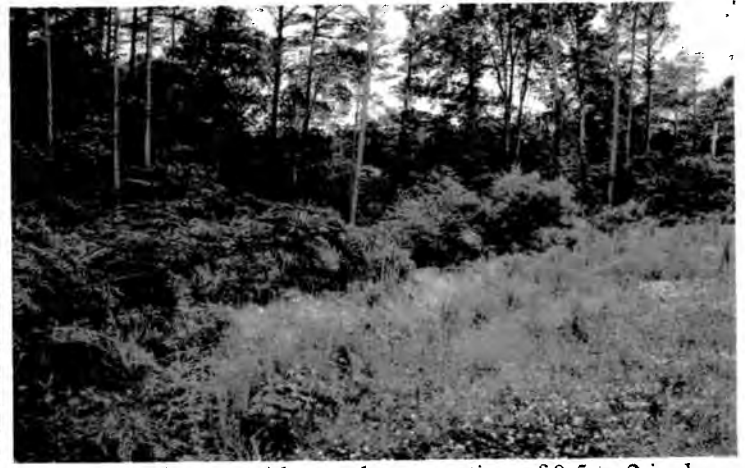
Basin embankment with woody vegetation of 0.5 to 2 inches
