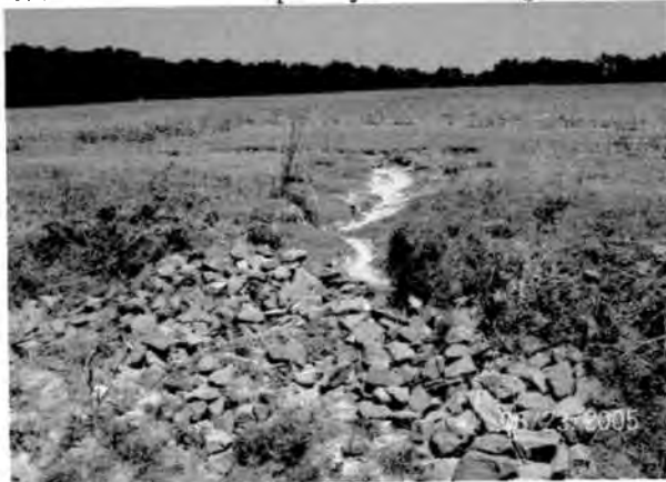
Erosion in watershed upstream of Basin inlet
