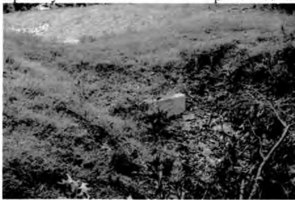
Properly vegetated downstream embankment w/minor erosion
