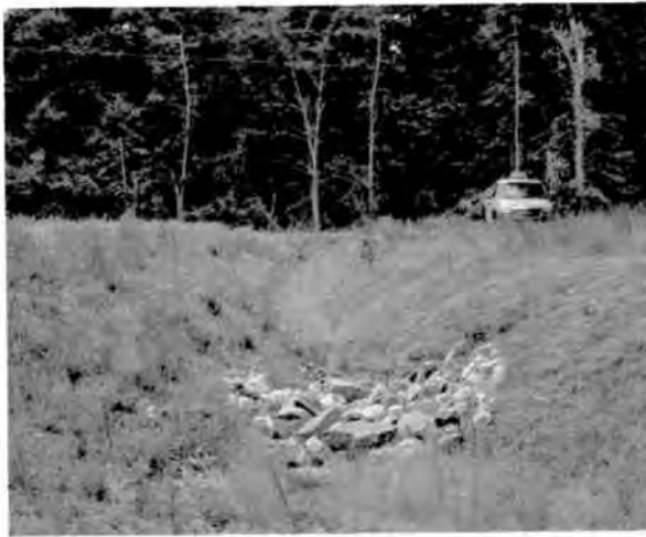
Stabilized conveyance channel into Basin
