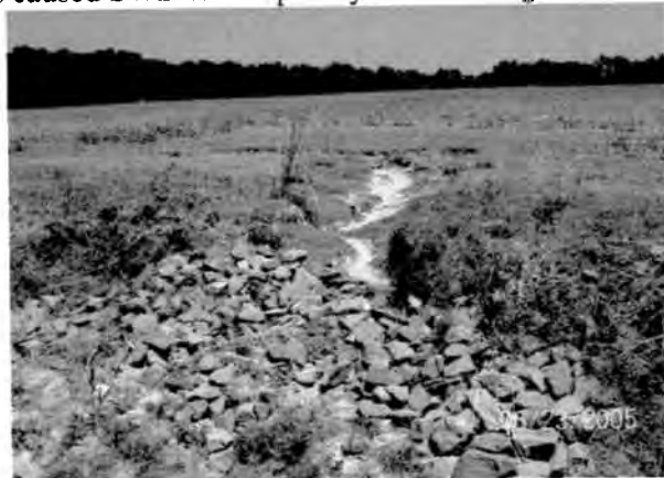
Erosion in watershed upstream of Basin inlet
