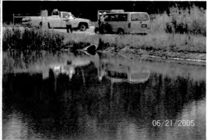
Principal spillway with pipe only, no structure
