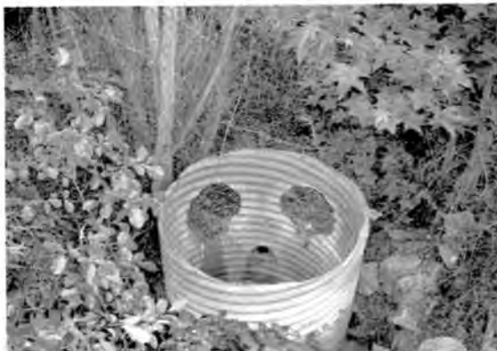
Functional & clear overflow spillway
