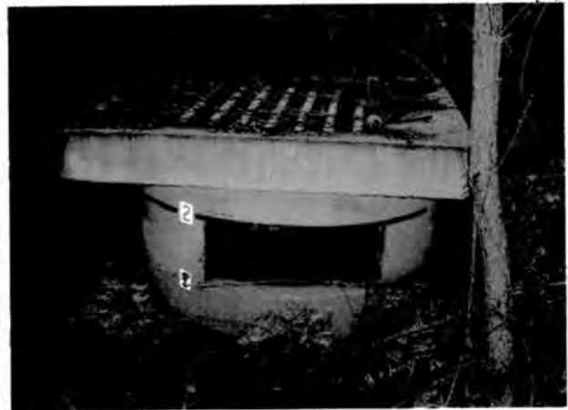
Clear low flow orifice w/ functional trashrack Low flow orifice blocked by trashrack
