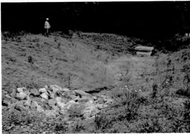
Well maintained and acceptable Basin embankment
