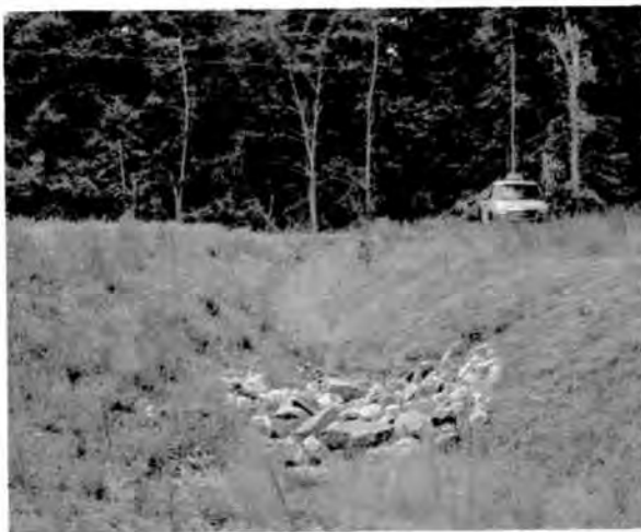
Stabilized conveyance channel into Basin
