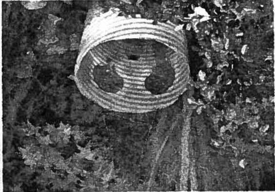
Functional & clear overflow spillway
