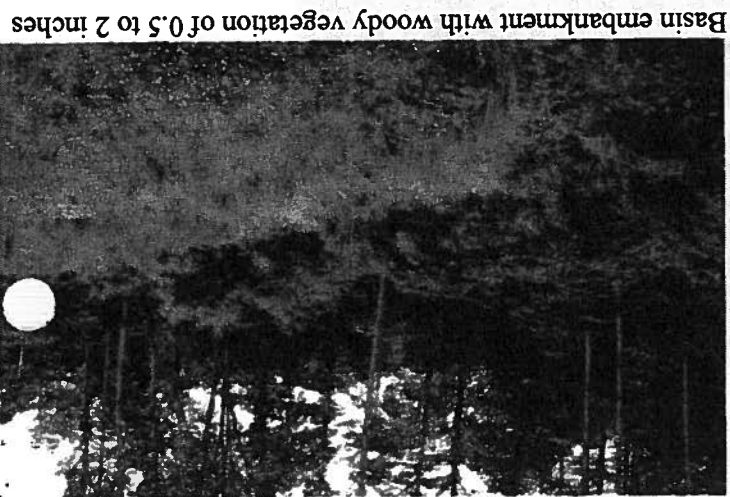
Well maintained and acceptable Basin embankment
