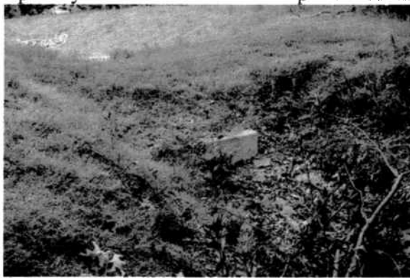
Properly vegetated downstream embankment w/minor erosion
