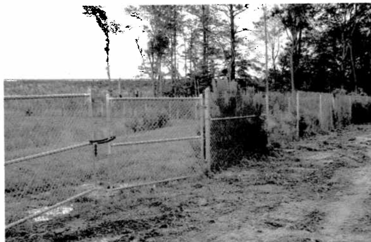
Fence surrounding Basin with gate unsecured and saplings growing in fence line
