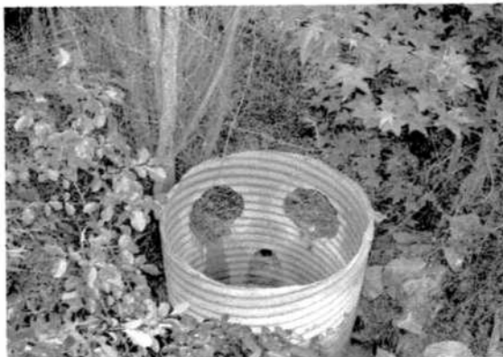
Functional & clear overflow spillway
