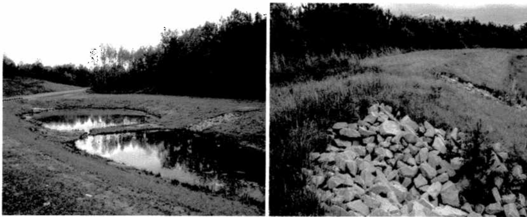
Good access to Basins as well as all the way around Basins for maintenance
