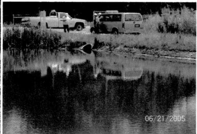
Principal spillway with pipe only, no structure
