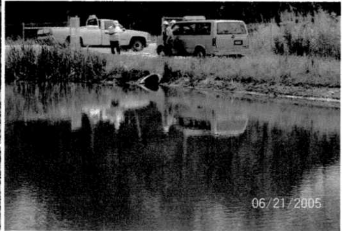
Principal spillway with pipe only, no structure
