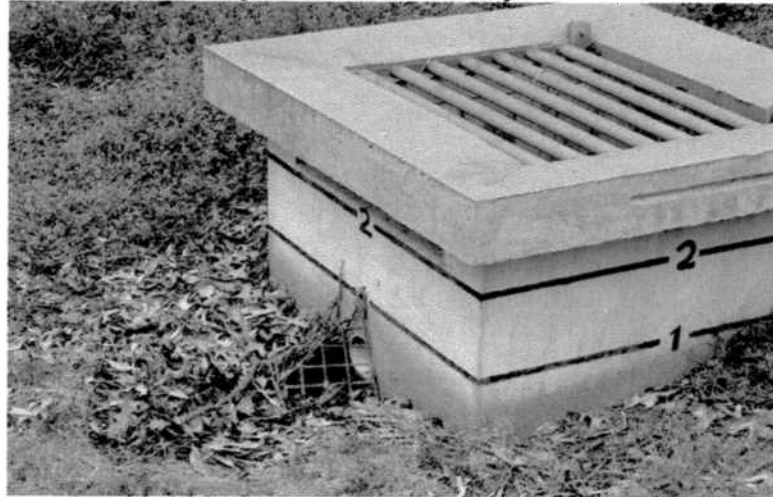
Trash rack clear and functional and structurally sound
