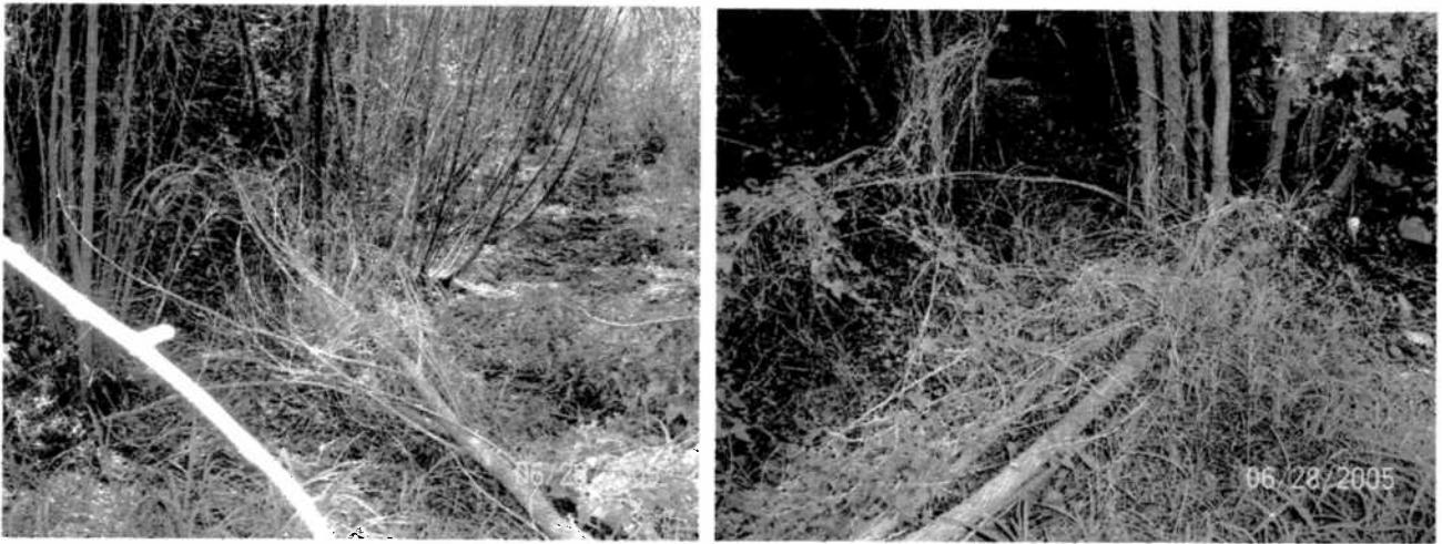
Fallen and dead woody vegetation can cause blockage in basin and possibly block outlet
