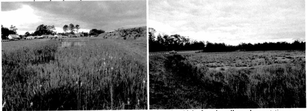
Shallow "Wet" basin with herbaceous vegetation "Dry" Basin with leafy and small woody vegetation
