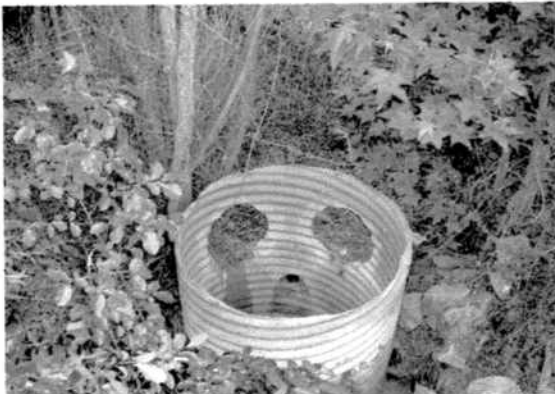
Functional & clear overflow spillway
