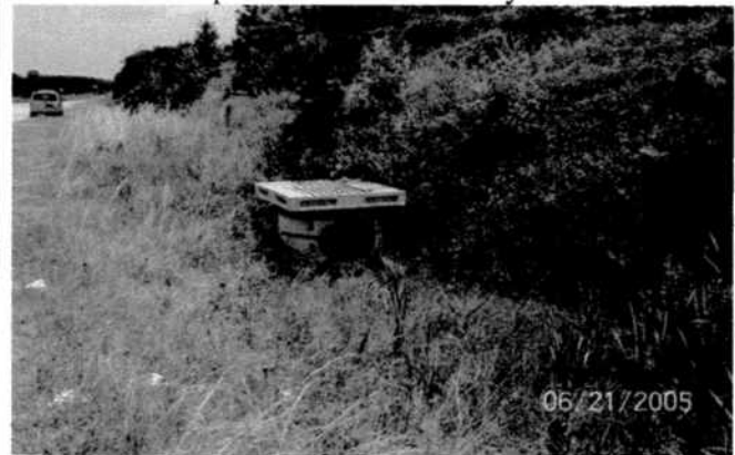
Clear & functional upper stage orifice
